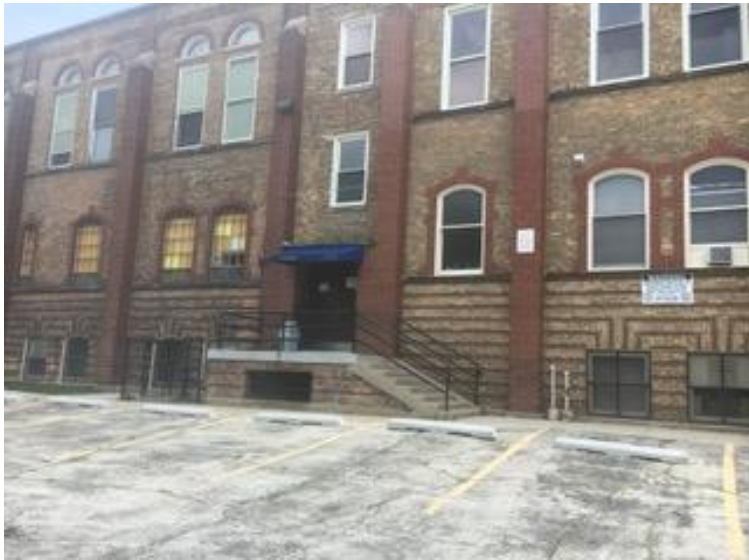
West Entrance from Parking Lot
